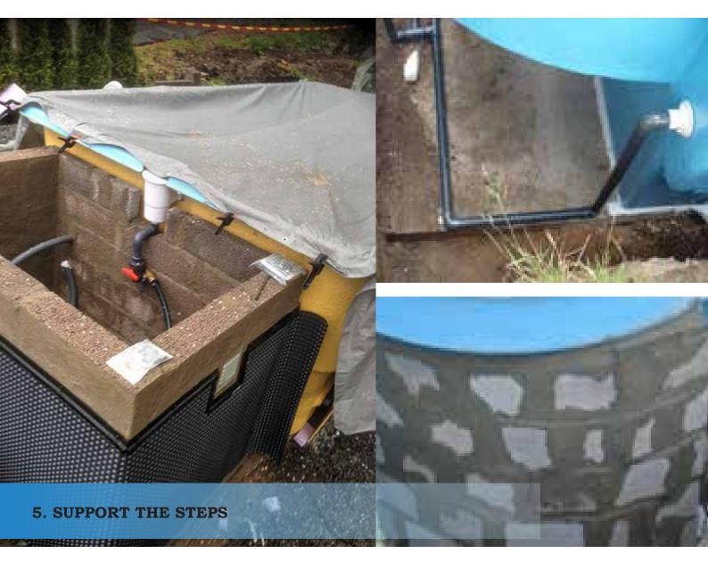
The steps should be supported with concrete blocks, properly checked for the correctness of their level. The fissure between the steps and concrete blocks should be filled with soft foam or it should be salienated all around. On the performed base plate we put the pool and make final checks on the level and the settings. After that we install the water system.
