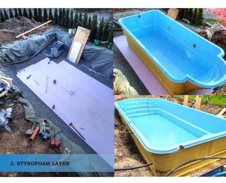
The foundation slab is a smooth mortar surface, any surface slopes shall not amount to more than 0,5%. All works should be consulted with a construction specialist well acquainted to local ground conditions. The swimming pool is to be placed upon the foundation slab, should it still possesses slight unevenness, the slab should be levelled with a styrofoam layer.
