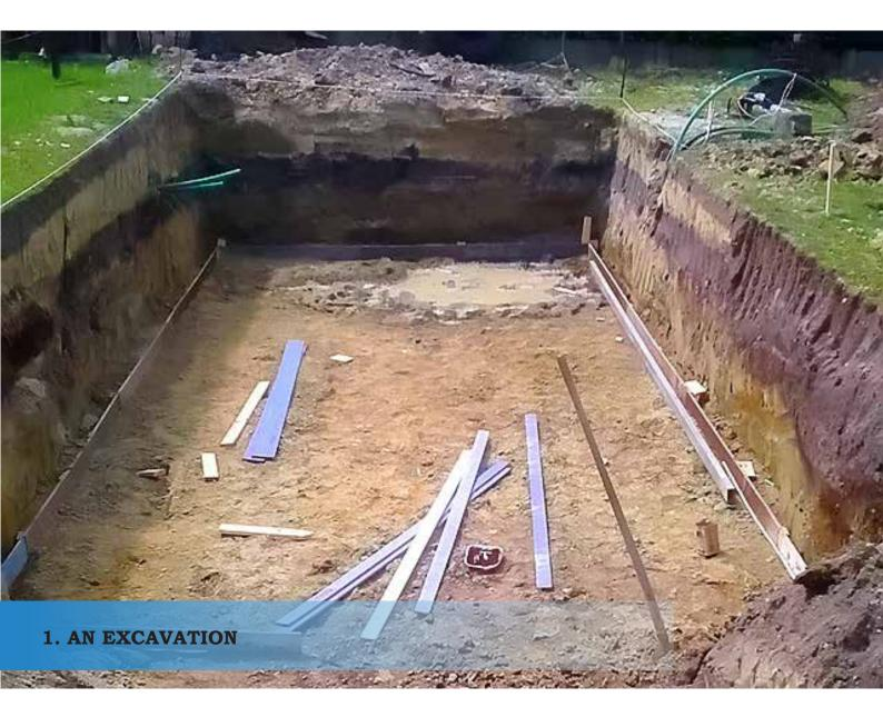
First construct an excavation pit in order to house the swimming pool taking into consideration the depth of the foundation slab. The size of the excavation pit constitutes the diameter of the swimming pool framework increased by 60-80 cm from each side – in order to ensure the proper conveyance of installation and piping works.
